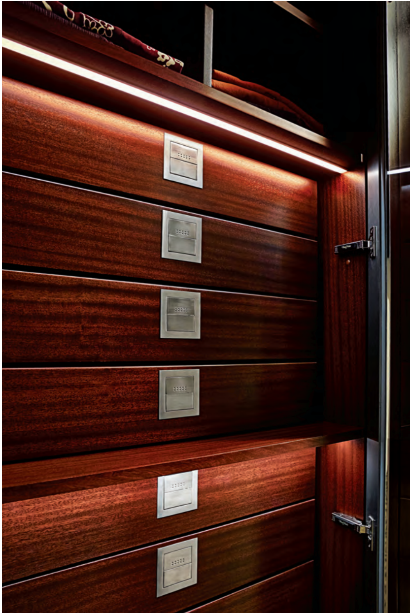
Fixed shelf lighting provides a wash effect on drawers below.
